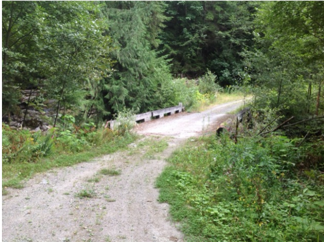
Approach from Right Bank when facing downstream
