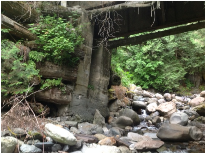
Right Bank Abutment when facing downstream
