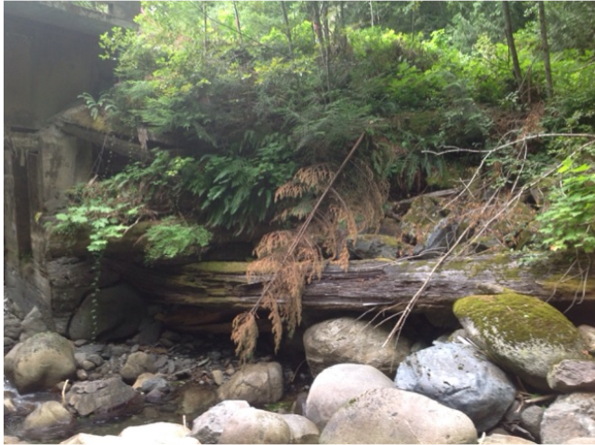
upstream right wing wall
