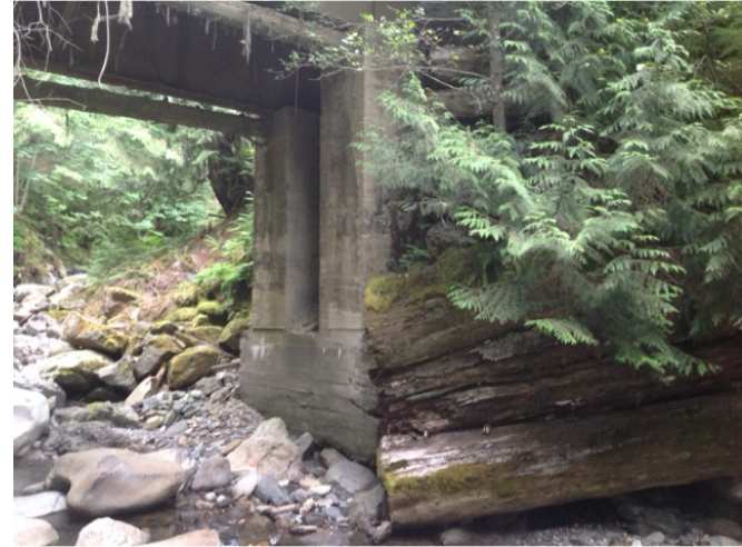
Left Bank Abutment when facing downstream
